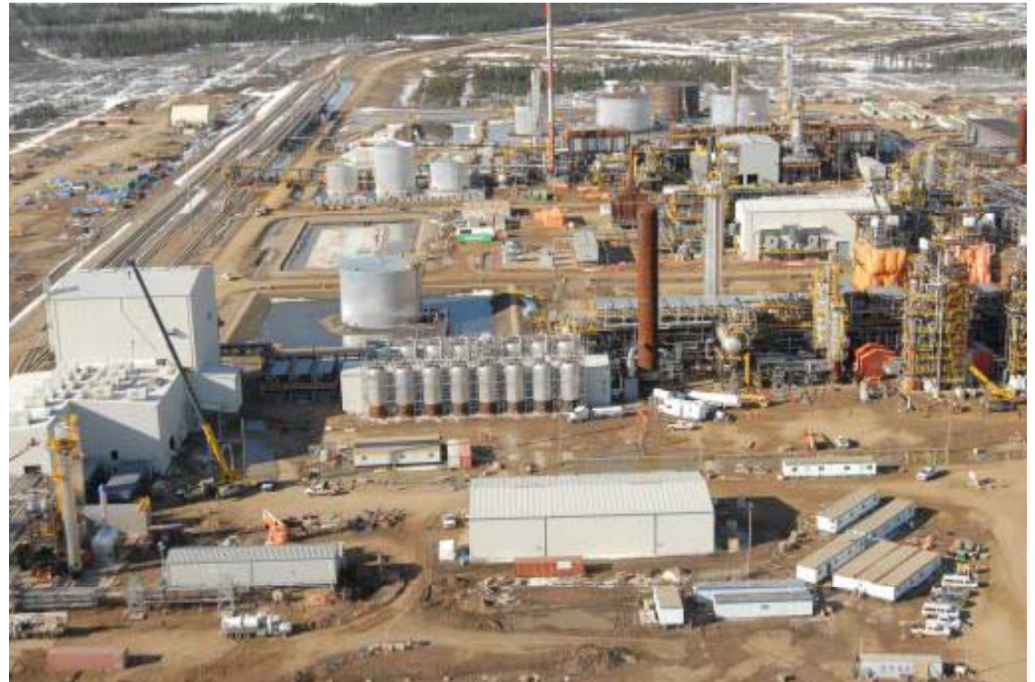
Nexen's Long Lake Gasifier, built by Flint in 2007
