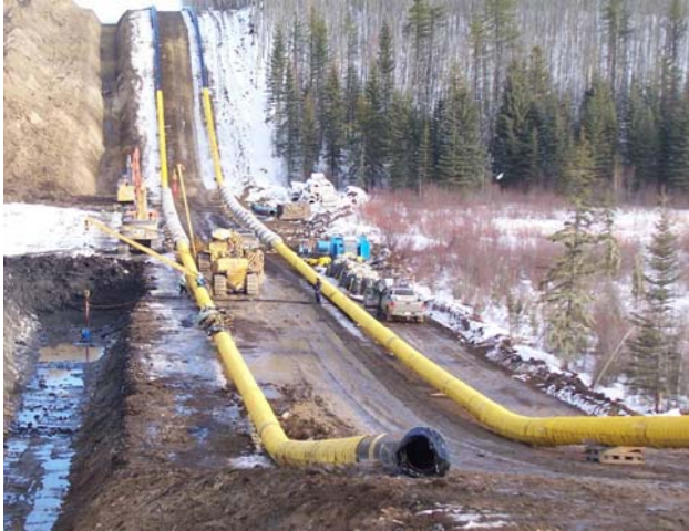
24 inch pipeline installation near Fort McMurray, AB
