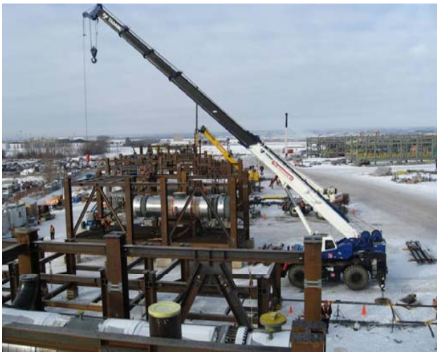
70 acre module fabrication yard, Sherwood Park, AB
